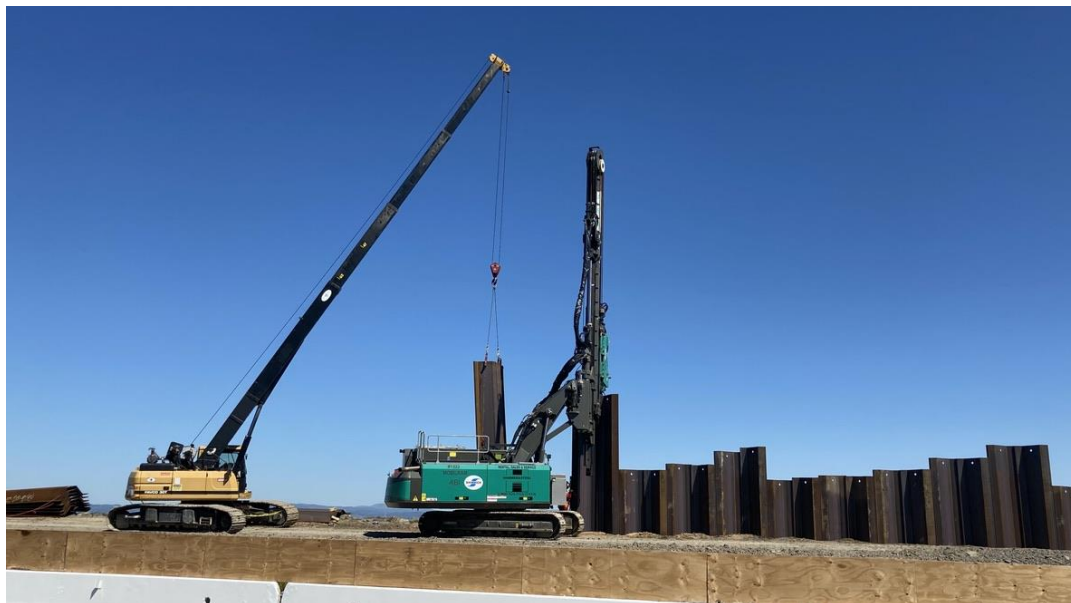
Foster City Levee upgrade, March 26, 2021 (Grand Jury photo)
